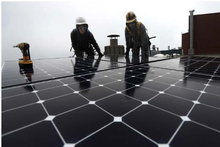
Workers install solar panels on the roof of a home on May 9th, 2018, in San Francisco, California. (Photo: Justin Sullivan/Getty Images)
